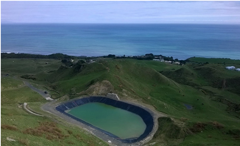
The newly constructed raw water storage dam at Mokau.
